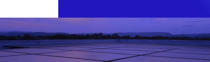
Application: HELIUP Stykon photovoltaic modules are designed for low-tilt waterproofing membrane roofs. The product is to be directly glued onto the new membrane during roofrepair. Its lifetime expectancy is matching that of most roof membranes making it the perfect tool to harvest energy from the sun.
